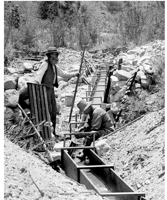
Placerita Canyon miners had to work hard to route the minimal water resources for sluicing.
