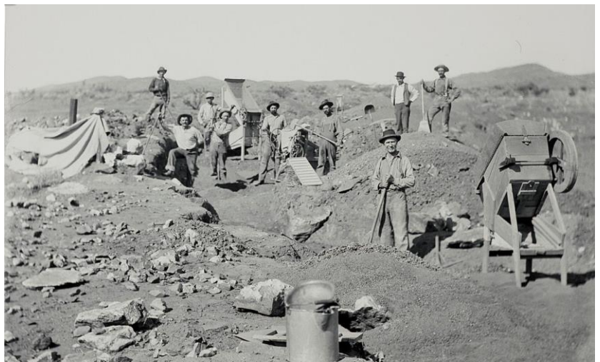
Dry washing for placer gold at the St. Elmo mine - Randsburg ca. 1897 Source: www.Westernmininghistory.com
