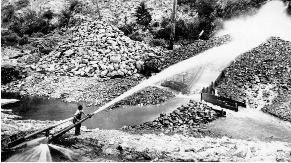
Hydraulic mining water cannon using high pressurized streams of water to process mass material that is then sent through sluices. Photo from UC California Archives
